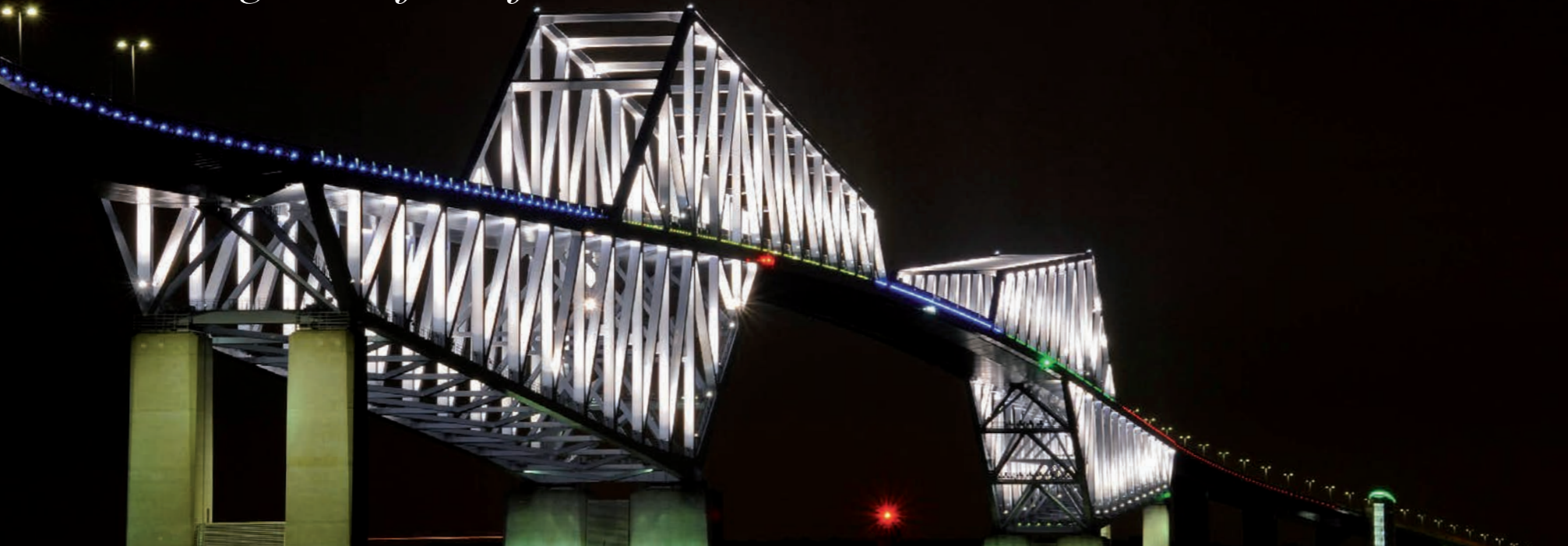
Tokyo Gate Bridge at night
