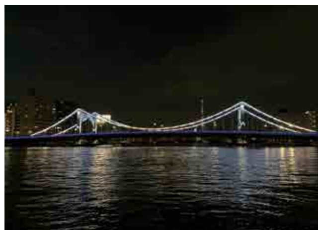
Kiyosu Bridge has been outfitted with a vibration-control system to protect against earthquakes.
