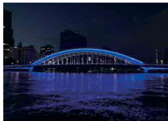
Rebuilt in 1926 after the Great Kanto Earthquake, Eitai Bridge has been equipped with bearings to dampen large seismic forces.
