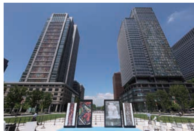
The sides of two massive skyscrapers became a pair of canvases. Each large-scale mural art had a distinct take on the theme, one of water and another of fire. Tokyo Tokyo FESTIVAL Special 13 “Super Wall Art Tokyo,” Drill Inc.
