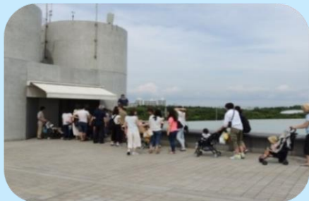
The waiting area for the elevator for visitors to enter is located outside the building, without roofing.
